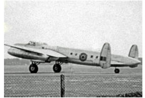
The Rolls-Royce Avro Lancasterian Nene test bed in 1948 fitted with the jet engines in the outboard position
