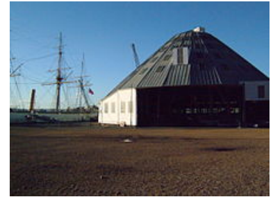
Slip 3 at Chatham Dockyard, designed and built by the Corps
