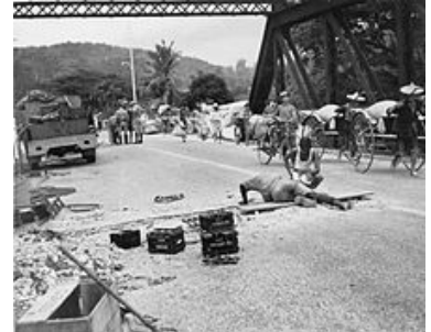
Combat Engineers prepare a bridge for demolition in Malaya.
