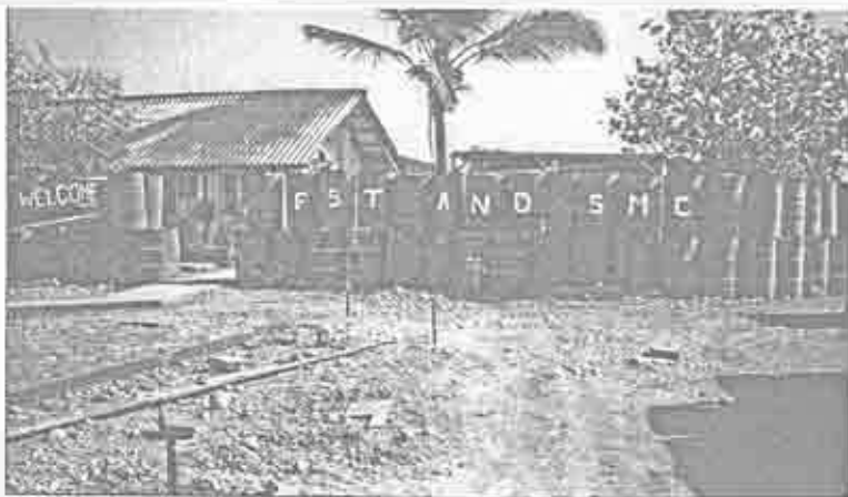
Above: The surgical team's oil drums are filled with sand, offering protection against small-arms fire and shrapnel.
